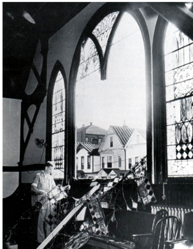
Hurricane Hazel destroys the main stain glass window in addition to parts of the roof (1954).
