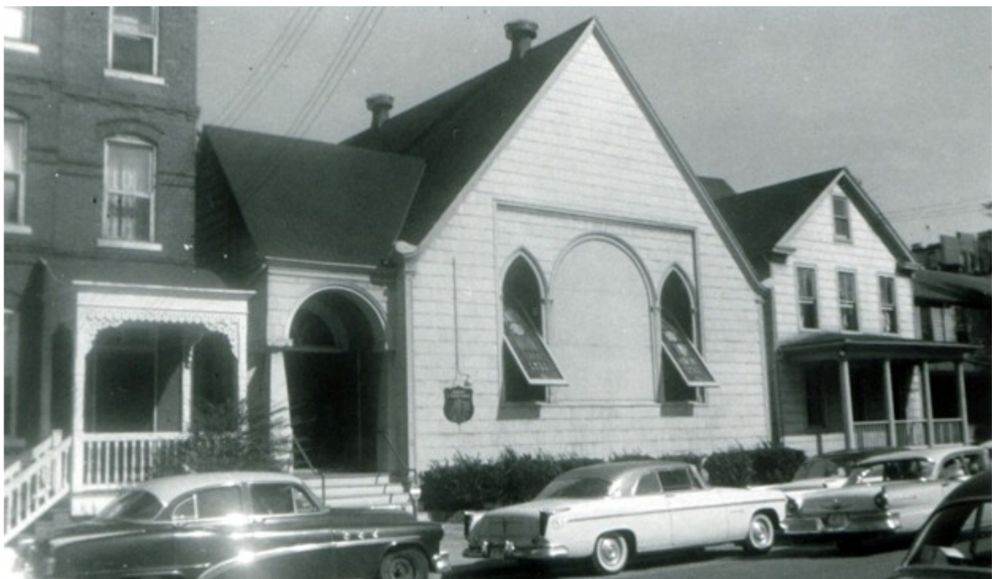
Trinity Lutheran Church following repairs as a result of Hurricane Hazel. This is how the Church looked in the days leading up to the final service on June 15, 1958. The building to the right of the Church was the Parish house.
